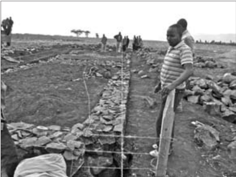
Determining the layout error of the foundation at the Gongali site.
