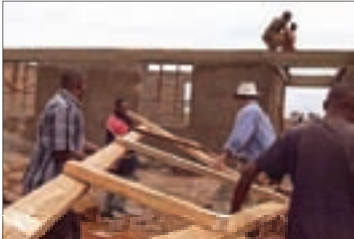
A truss ready for hoisting.
